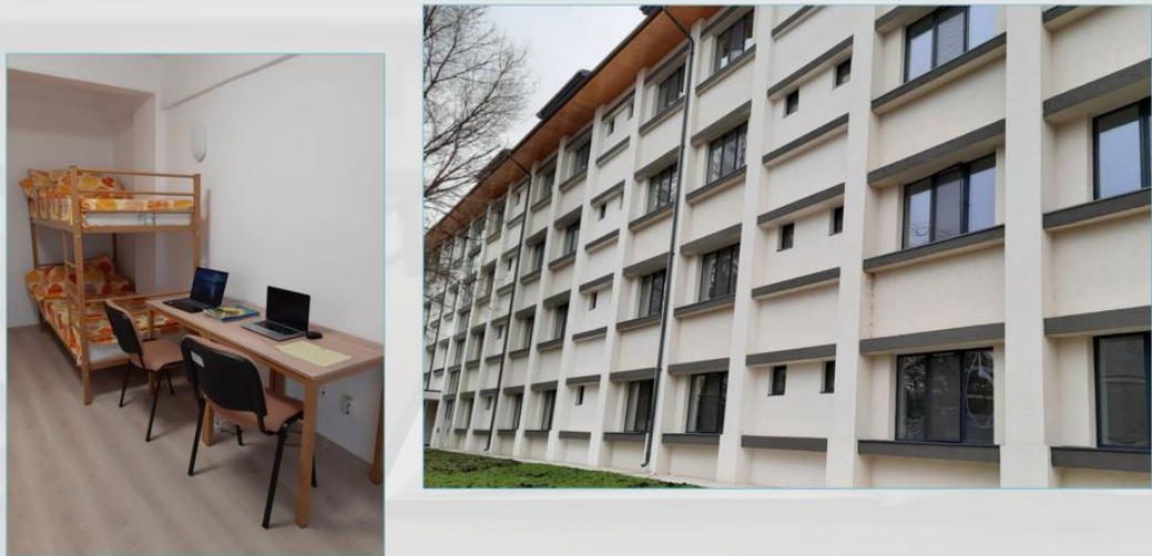
SCHOOL BOARDING FACILITY
